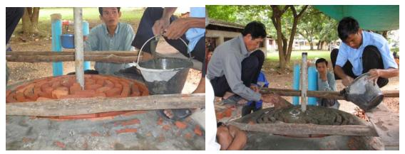
Once the construction of brick work and fixation of main gas pipe completes, the outside of the dome should be flushed with cement water slurry using a broom or brush. This Plain cement flush (1 cement: 3 to 5 water by volume) should be well sprinkled on the surface to close any cavities left while constructing brick dome.
