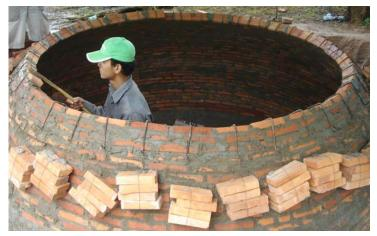
■ When construction of wall reaches in the stage that the diameter of the top hole is about 50-60 cm, it is difficult to construct wall with brick and counterweights. To construct this portion, scaffoldings are provided from the bottom inside the digester, to support the wooden planks as frameworks. Soil in the shape of top of dome is prepared as mould for laying bricks in this part. Sand is sprinkled in this mould before laying brick and compacting with mortar.
