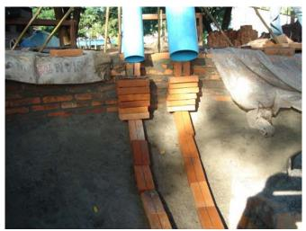
When the height of wall reaches equal to height of manhole as shown in the drawing, arch for manhole has to be constructed with the help of framework. Bricks should be placed in either side as support and a horizontal plank should be placed above the brick support. To maintain a dome shape, soil has to be placed above the plank at the desired shape. Brick has to be laid on edge maintaining the inner curvature of wall with the help of guiding bamboo.
