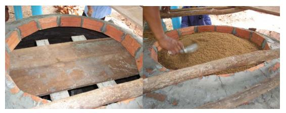
Main gas pipe has to be fitted in the centre of the dome while constructing this part of gas holder. 60 cm long GI pipe of 3.5 cm diameter with reducing elbow (3.5 cm to 1.5 cm) in one end is used as main gas pipe. The other end of the pipe consists of welded MS rods 3 numbers of 10 cm long and 8 mm dia to ensure firm stability of the pipe. This end is properly fixed and concreted in the dome.
