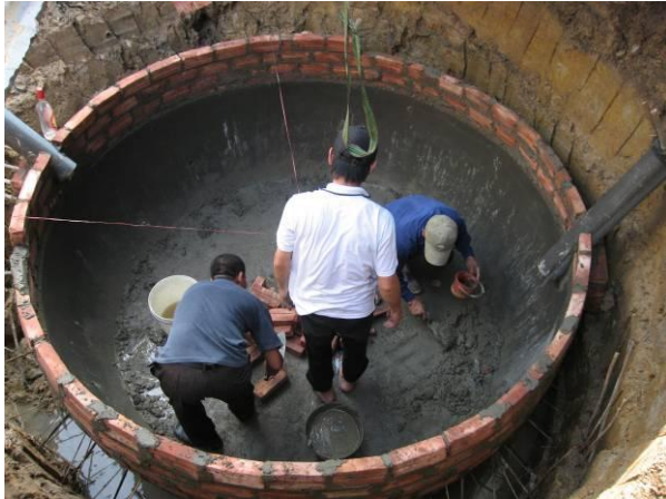
Figure VI-12: Some pictures of construction of KT1 (excavation, construction of wall, plastering)
