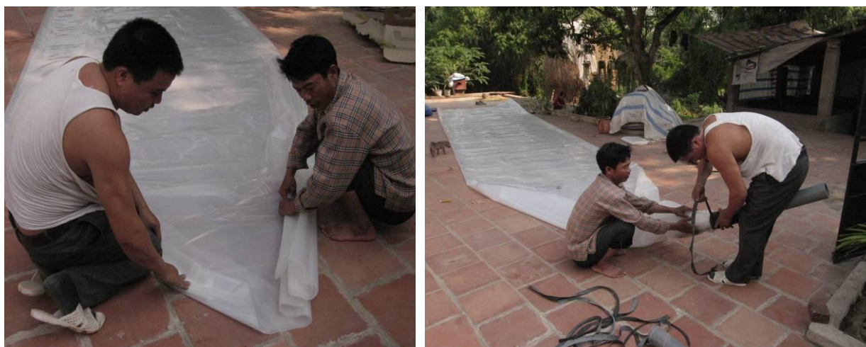
Figure VI-9: Installation of inlet and outlet pipes
