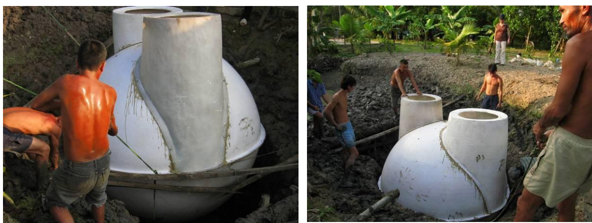
Figure VI-6. Lowering composite digester
