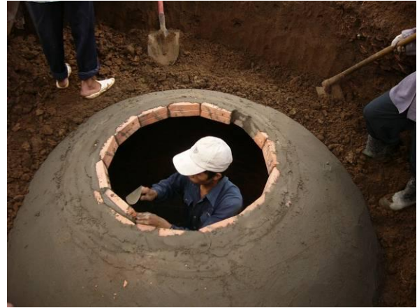
Figure VI-12: Some pictures of construction of KT1 (excavation, construction of wall, plastering)
