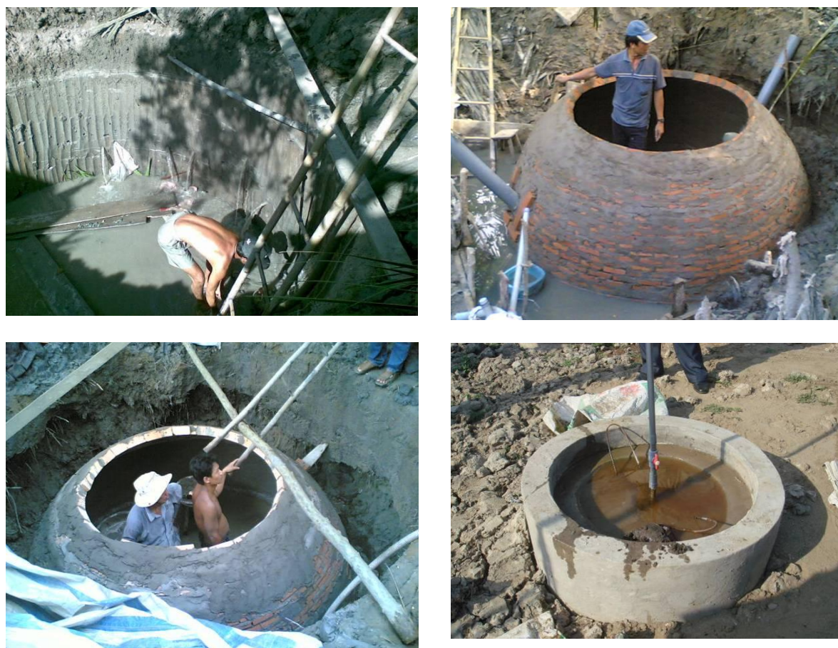
Figure VI-13: Some pictures of construction of KT2 (excavation, construction of wall, plastering)
