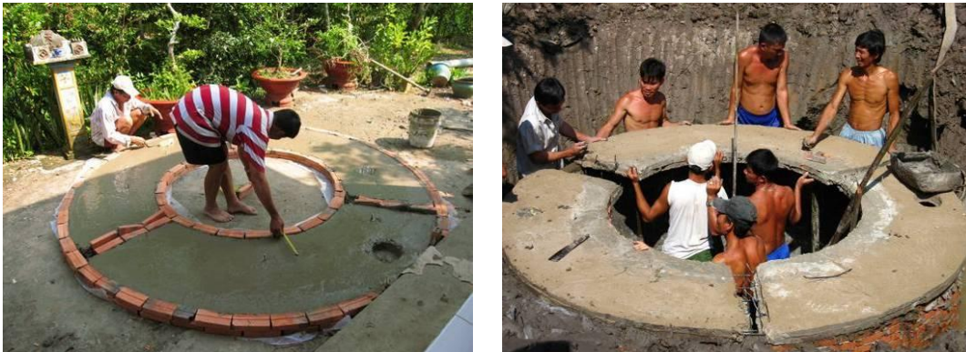
Figure VI-3: Concrete to separate digester and compensation section in Hanoi
