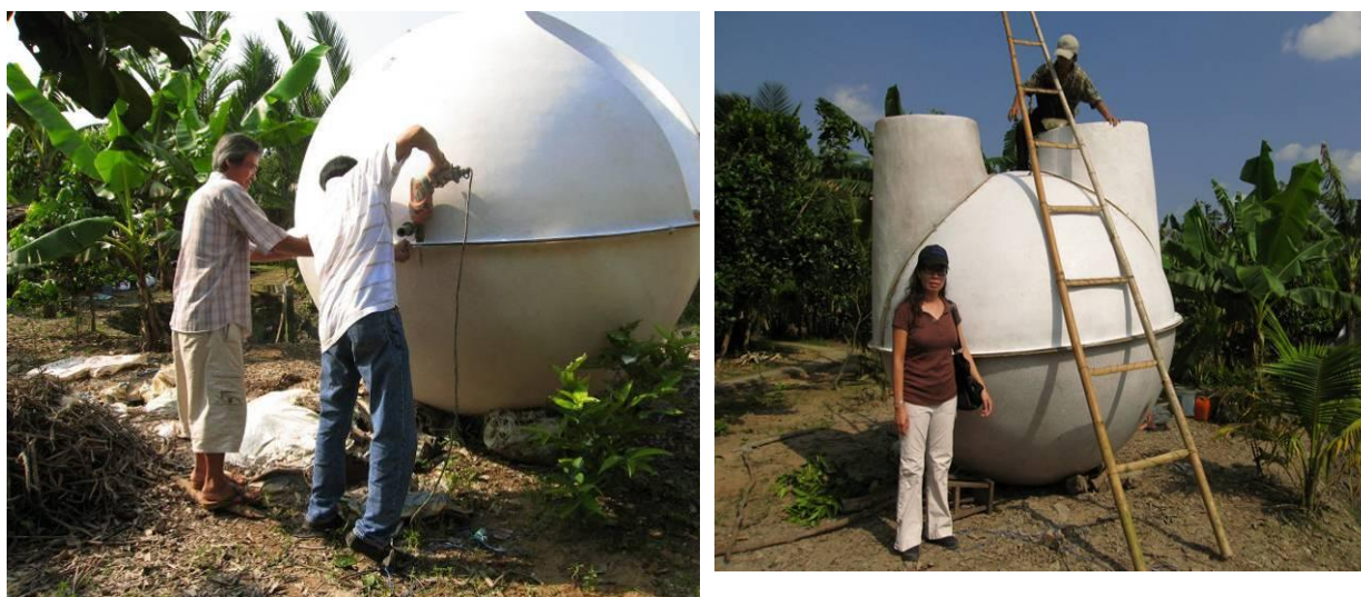
Figure VI-6. Lowering composite digester
