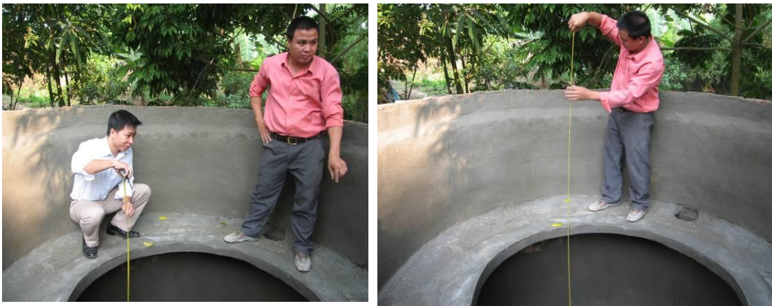
Figure VI-3: Concrete to separate digester and compensation section in Hanoi
