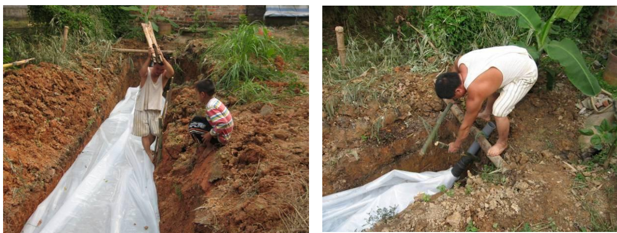
Figure VI-10: Putting nylon bag digester into hole
