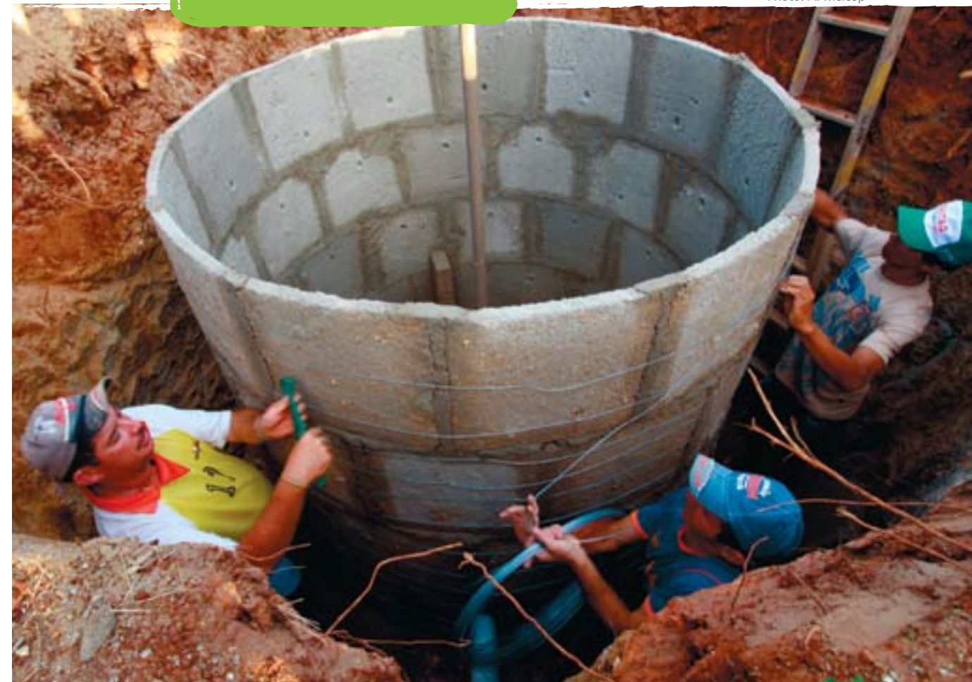
[Figure 14] Tying the wall with galvanised wire
